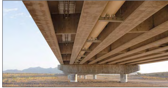
A portion of the Gilbert Road Pipeline is secured underneath the Gilbert Bridge that crosses the Salt River. Photo courtesy SRP.
