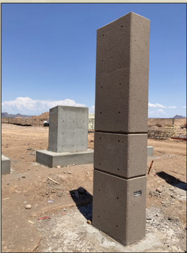
Memorial shade structure column in foreground with service branch column in back.
