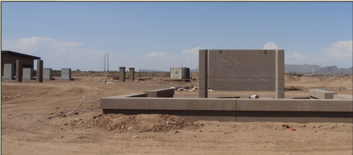
Committal shelter structure and seating area progress.
