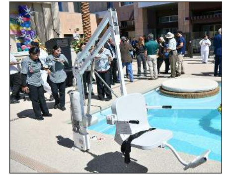
One of the ADA-approved chairs installed to increase accessibility to the new pool.
