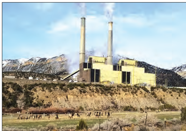
Huntington Power Plant
