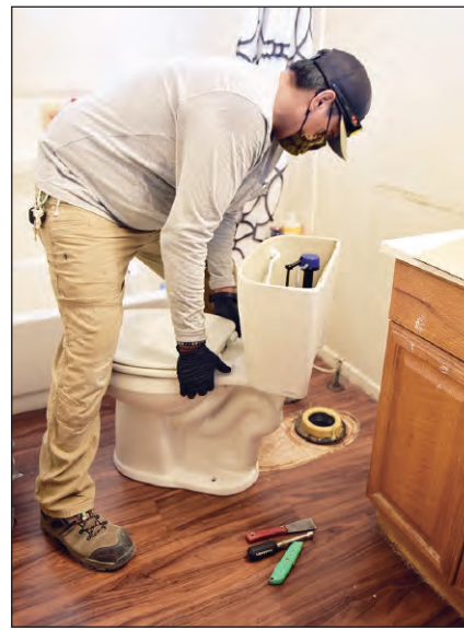
Foster begins to place the new toilet for its final installment.
