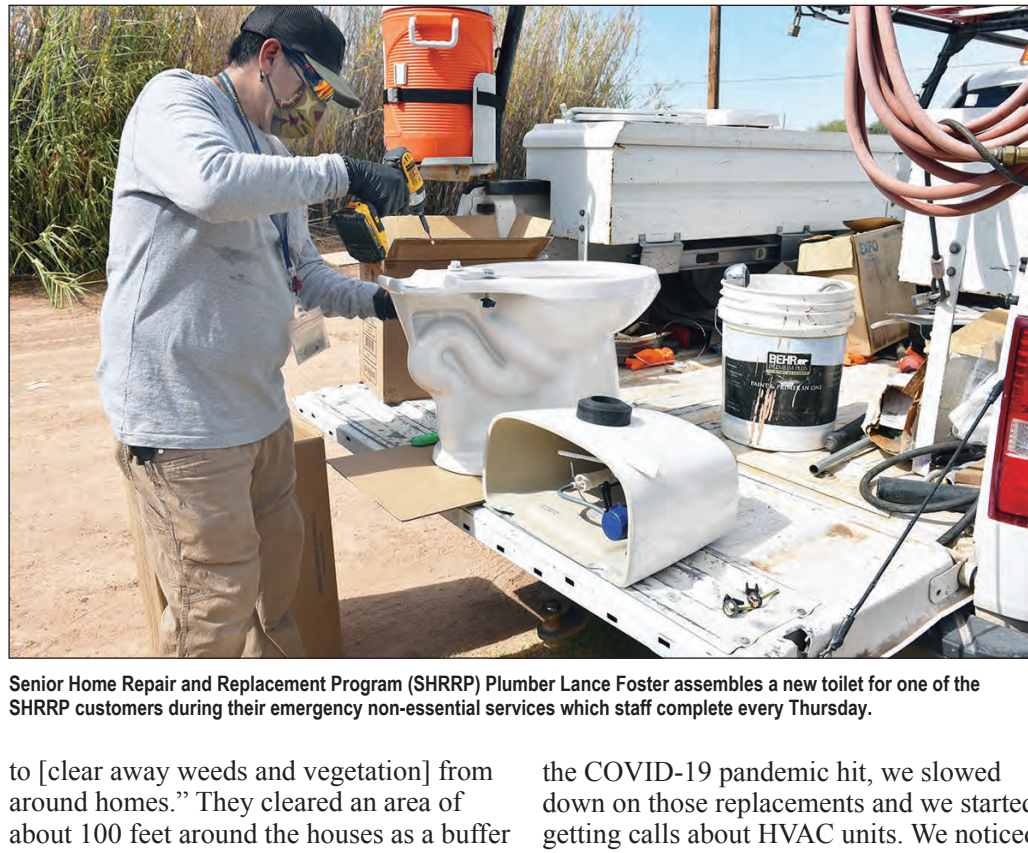
Senior Home Repair and Replacement Program (SHRRP) Plumber Lance Foster assembles a new toilet for one of the SHRRP customers during their emergency non-essential services which staff complete every Thursday.
