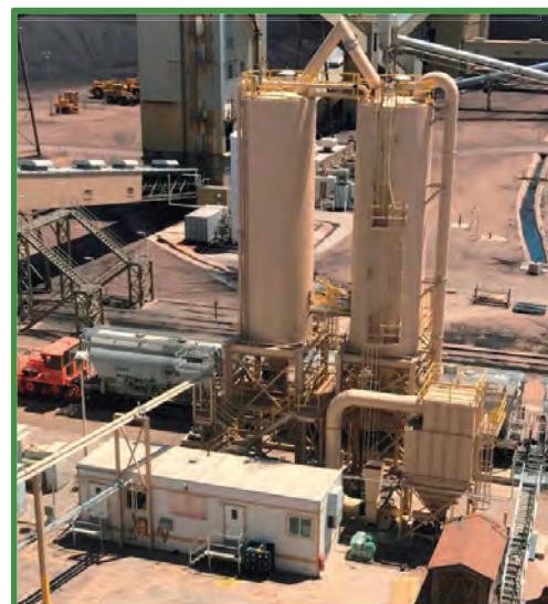
Rail Load Out and Storage Silos
