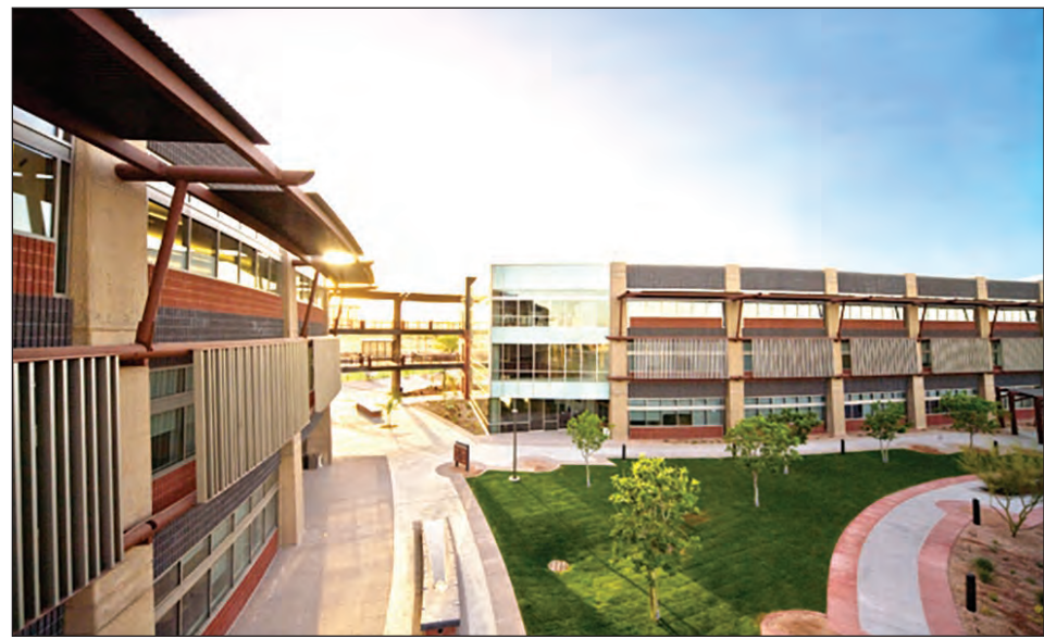
Two Waters Tribal Complex, one of the many projects Auger was a big part of. Photo provided by Harold Jones
