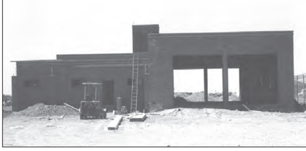
Salt River Fire Station 291 under construction. Photo was taken approximately 1981.
