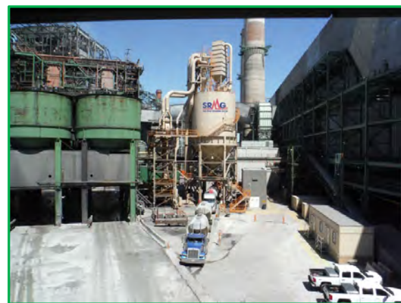
SRMG Four Corners Fly Ash Beneficiation Facility
