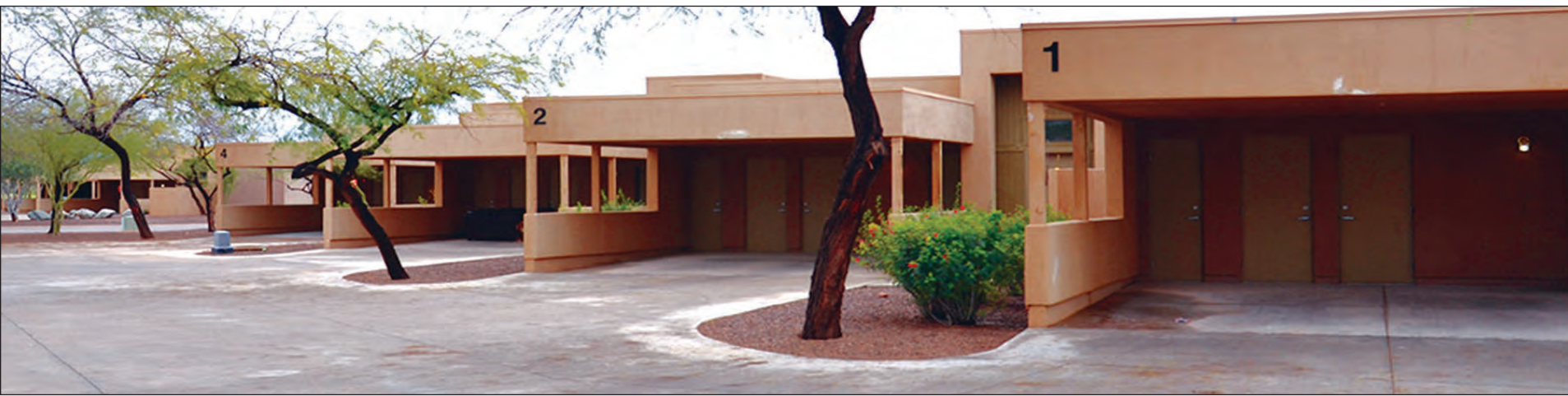
PAL Program apartments current housing that will be renovated for SRPMIC Housing.
