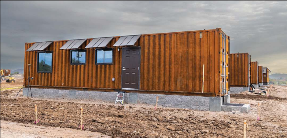
An exterior view of the transitional housing unit, is made of refurbished Conex boxes that have been modified into fully insulated living spaces.
