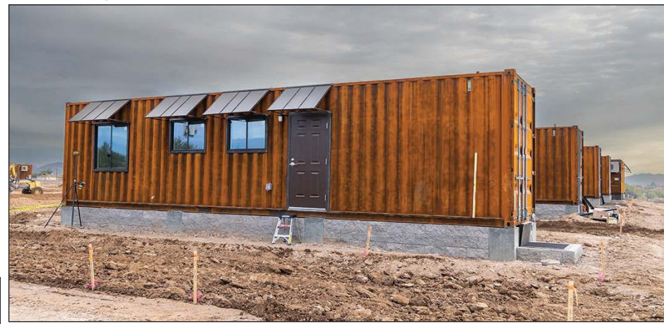
An exterior view of the transitional housing unit, is made of refurbished Conex boxes that have been modified into fully insulated living spaces.
