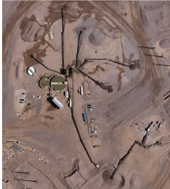
Crusher at Beeline Plant
