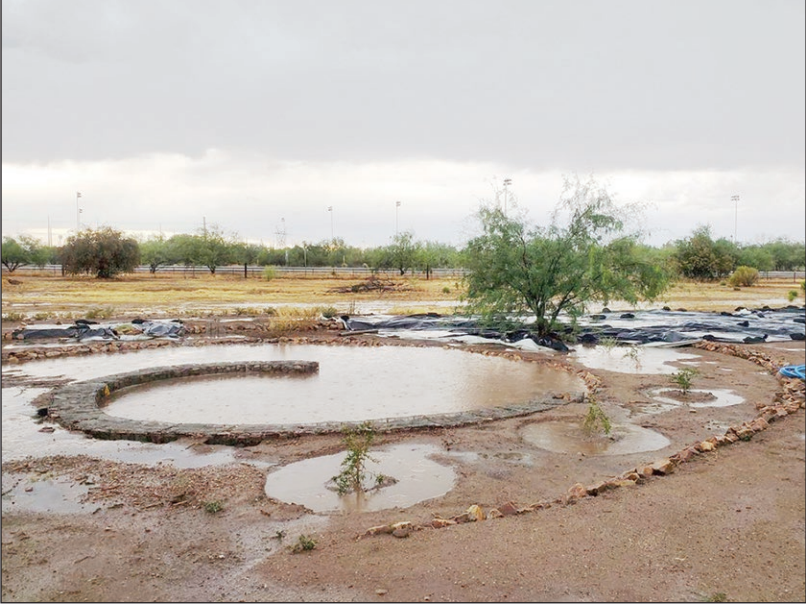
The spiral basin, which is at the end of the parking lot at the Native Seeds/SEARCH Conservation Center in Tucson, serves as an area for overflow from the existing basins to infiltrate the soil. Photo courtesy of Native Seeds/SEARCH
