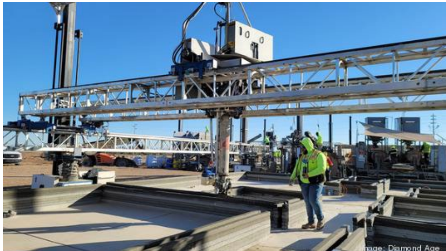
This construction automation system can leverage 3D printing to build homes in less than 60 days.
