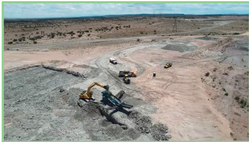
Excavating Landfilled Fly Ash
