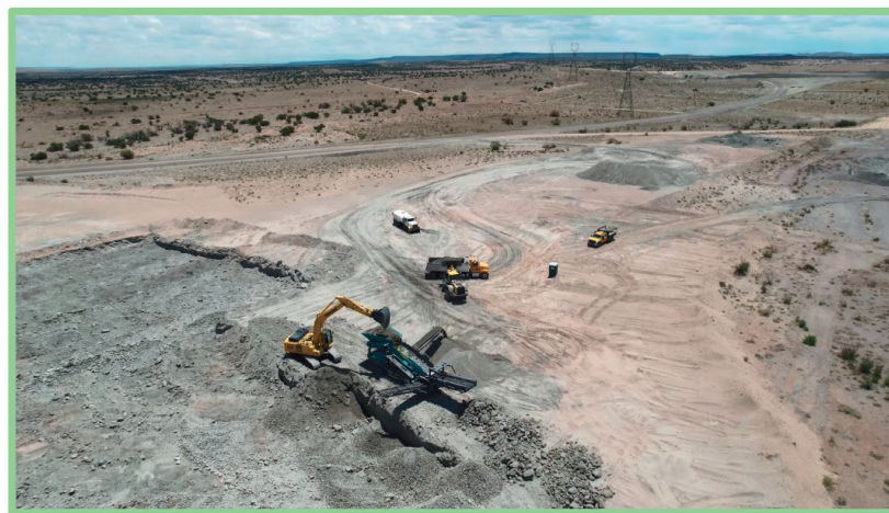
Excavating Landfilled Fly Ash
