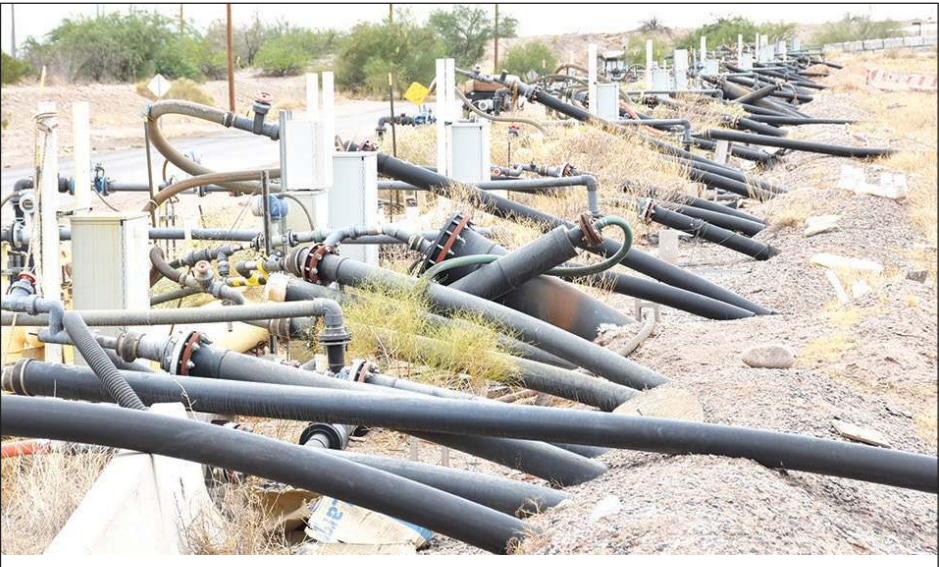
Pipes that collect gas from decomposing waste at the Salt River Landfill.
