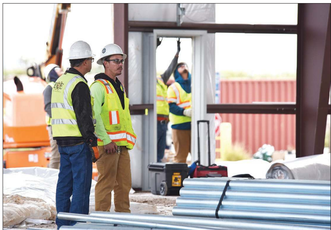
Workers begin to construct the doorways to the new recycling facility.
