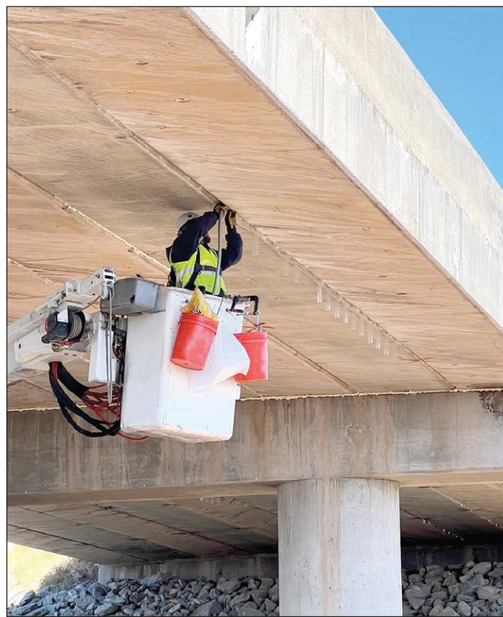
Bat Mitigation. Photo courtesy of Maricopa Department of Transportation
