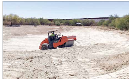
Construction crew continues replacing the old lining of Quitobaquito Pond. Photo courtesy of the National Park Service
