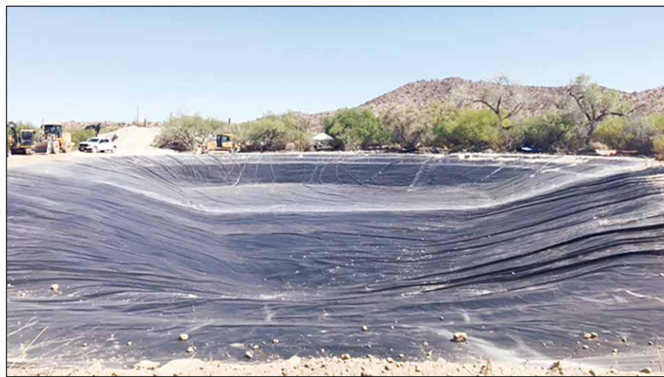
New lining being inserted in the Quitobaquito Pond at at Quitobaquito Springs at Organ Pipe Cactus National Monument. Photo courtesy of the National Park Service
